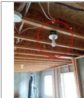
Exposed wires
